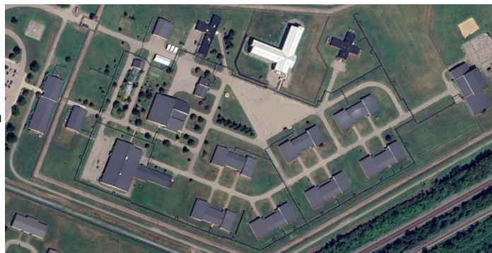
Aerial View of Facility with New Overhead Piping Visible Throughout
