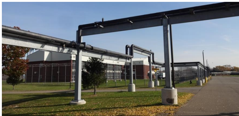
Overhead Piping Installation
